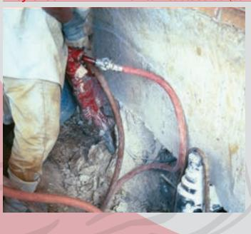
depth of 15' below grade. The shafts were designed to support suspended grade beams cast on carton void forms. Testing determined that deep seated heave was occurring which was actually lifting the drilled shafts, in turn lifting the perimeter grade beams. The heave resulted due to no provisions being made to drain the select fill.
