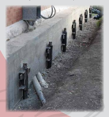
transfer the foundation loads to the piles, Messrs. Cutler and Gallaway developed a plan utilizing two concrete beams that were dowelled to the existing limestone footing and cast parallel to the existing footing. This was the same system that had been implemented previously with great success. The footings were cast with pre-manufactured embed pile brackets that received the steel piles.
