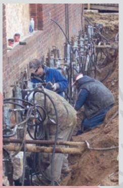
The high loading of the perimeter spread footing required that helical piles be spaced 3' 6" apart, and would need to develop high capacities. Of particular interest, this job required that all piles had to be lifted simultaneously to prevent damage to the historic masonry exterior. This was easily accomplished by utilizing Power Lift's patented synchronized lifting system. The building was lifted and the footing was permanently re-supported with Power Lift Helical piles.
