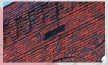
it later became the McAdoo Hotel and served as housing for returning servicemen in WWII. Over time, differential movement occurred due to consolation of the highly plastic clays, causing distress in the exterior walls.
